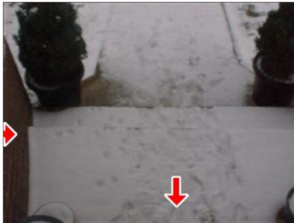
2.3 Picture 1 Photo of steps at entry.
