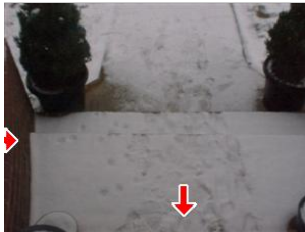
2.3 Picture 1 Photo of steps at entry.
